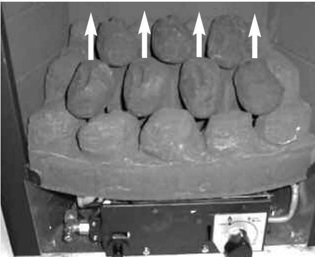
The exact position and fit of the coals may be finely adjusted to give the best appearance.
